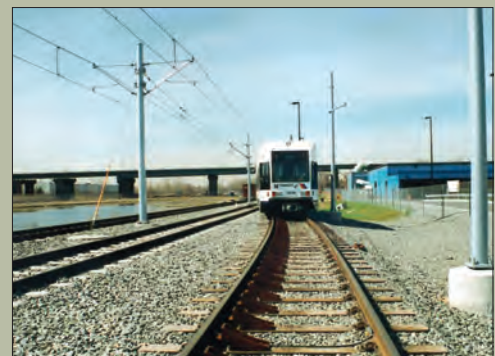
(from top) Air Train Jamaica Station, Queens, New York; Alameda Corridor, Los Angeles, California; Hudson-Ber- gen Light Rail Transit DBOM, Bayonne to Hoboken, New Jersey
